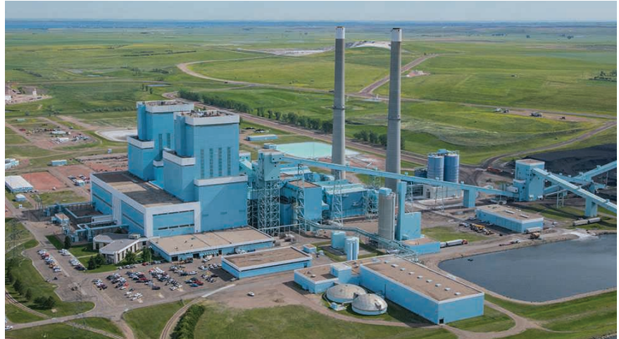
The Antelope Valley power plant near Beulah is capable of producing 900 MW of electricity.
