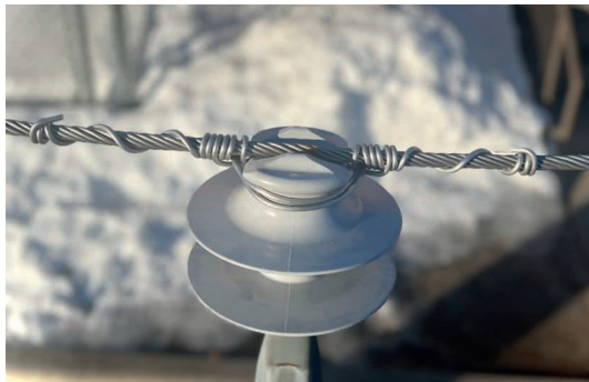
Newly tied conductor on an insulator
